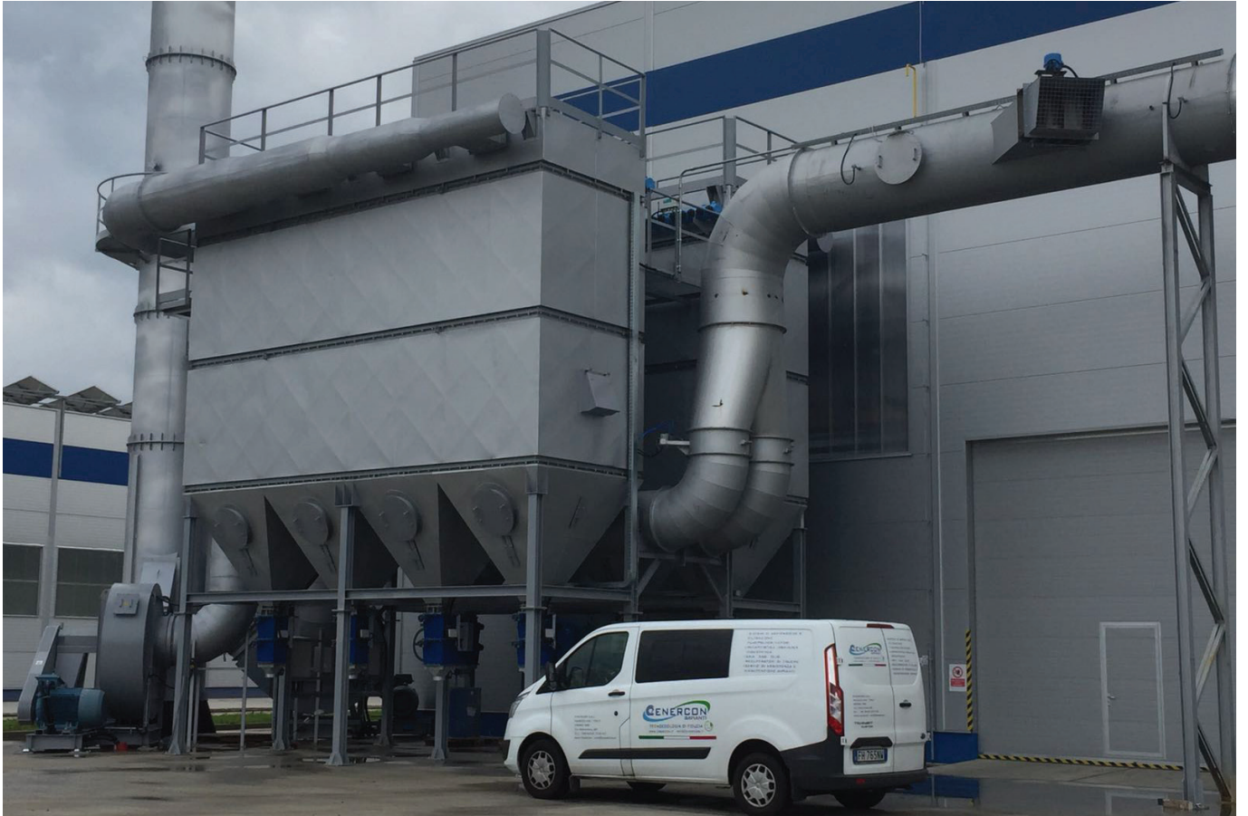
■ 85,000 m 3 /h suction and filtration system for fumes treatment from aluminum melting furnaces - Slovakia
