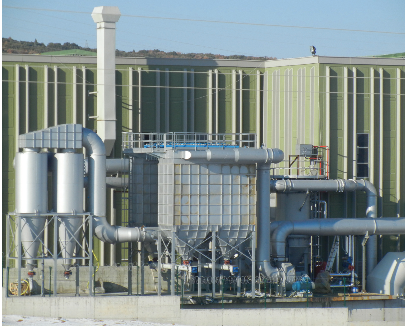
■ Fume suction and filtration technology systems from melting furnaces complete with fume/water heat exchanger for aluminum foundry - Turkey
