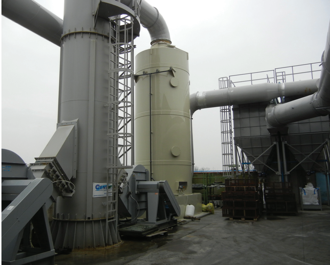
■ Technological systems for suction, dust filtration and odor abatement from bronze shell casting machines and bronze melting furnaces - Italy
